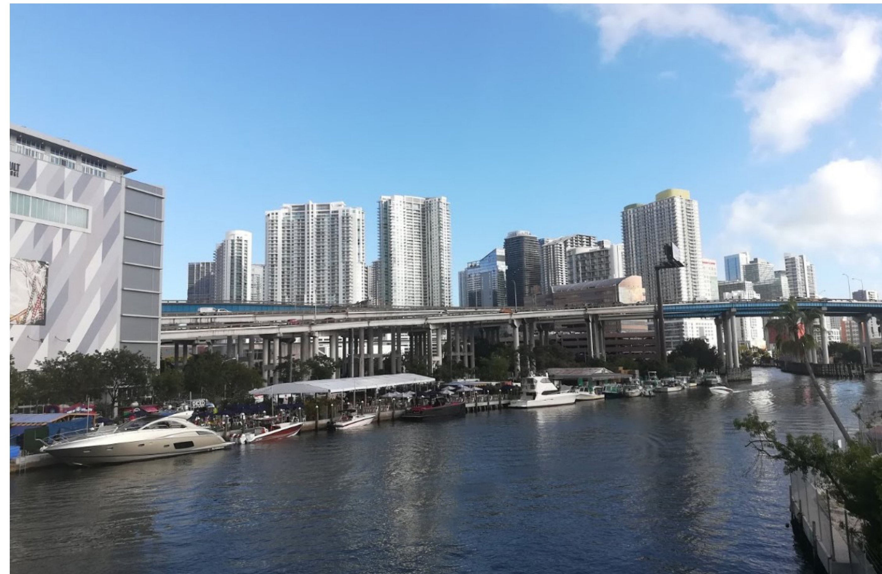
F View C - Looking from Bridge on SW 1st St.
